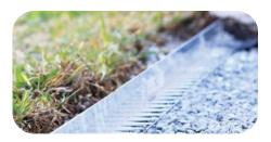
1. Shape Formation – Create the desired shape using border systems (aluminium, Corten steel, wood, or plastic) with a height of 5-15 cm, depending on load requirements.
