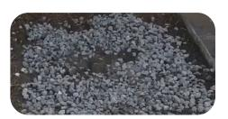
2. Create a Level Base – Spread a 5–7 cm layer of mixed sand and crushed stone. Ensure the surface is leveled at a minimum 3° incline for proper drainage. Install BERA® Edging Systems to secure the borders.
