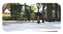
**4. Laying the Sheets** – Align sheets by overlapping the geo-textile lips for stability, weed control, and support.
